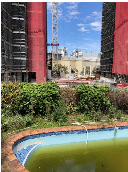
Picture 3 - Looking South from 7 Gray Street on-site
