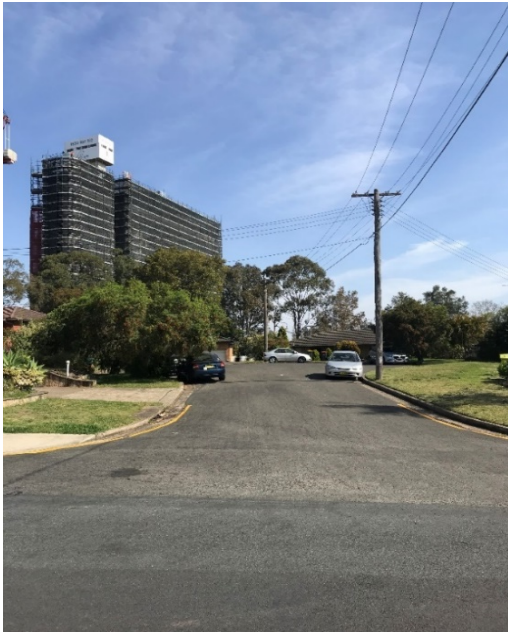
Picture 1 - Looking South Towards Vivien Place from Gilham Street
